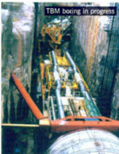
riverbanks. The only feasible method to control the flood was to tap the water upstream and divert part of the water before it entered the critical area. A large tunnel (11.83 m inner diameter, 9.7 km-long) was required to store and divert the floodwater. Thus, the ambitious SMART Project came into existence.
