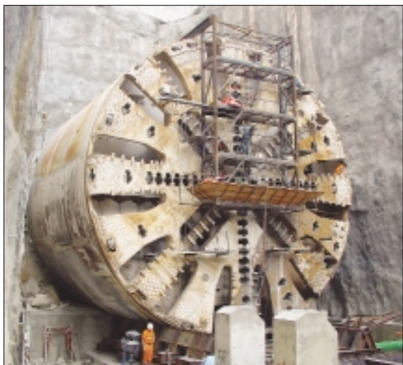
▲ Tough Cut. Tricky ground conditions required slurry-pressure TBMs.
