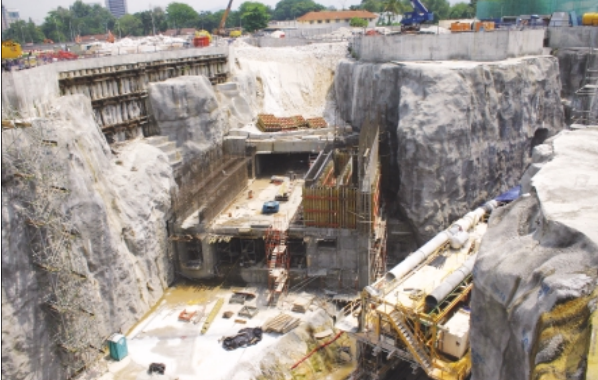
▲ Junction. Contractor had to haul TBM through huge open pit excavated to accommodate highway connection.
