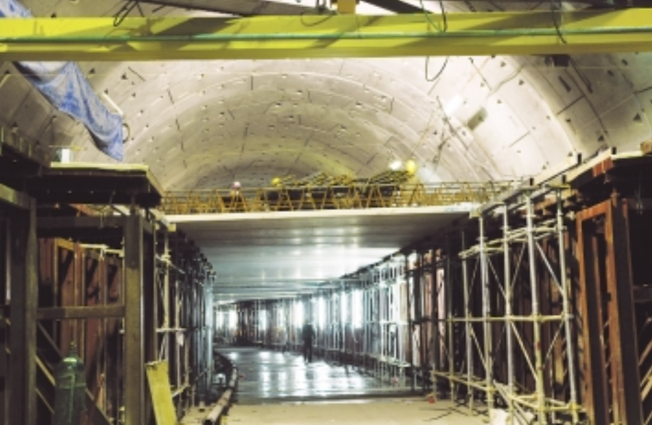
▲ Double Deck. Highway decks are attached to lining segments with shear connectors.
