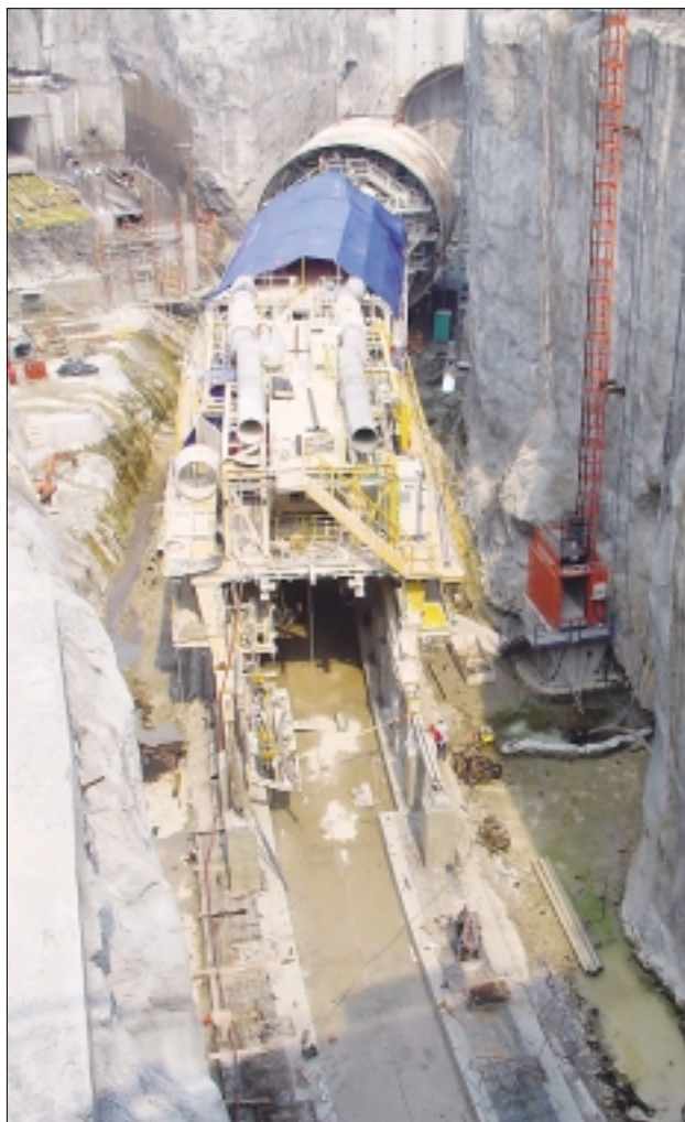
▲ Curves. Tunnel has tighter bends than normal for a large TBM.
