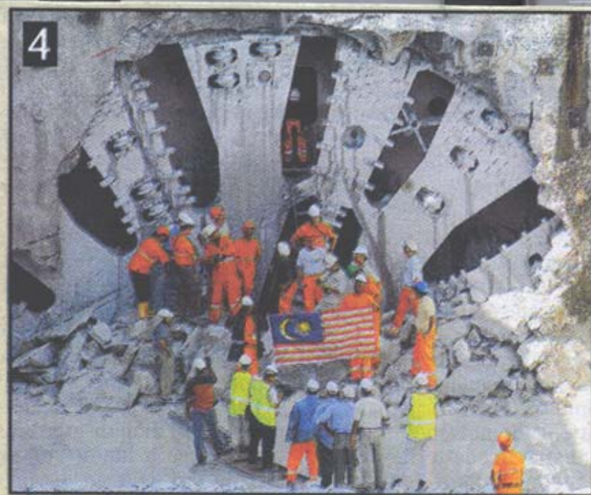
BREAKING OUT: (from top) Tuah , the giant boring machine, emerging through the ground yesterday to an excited reception from workers at the site. — Pictures by Amirudin Saib
